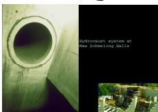
At the MSH we re-invented an ecological heating system over 2000 years old, the hydrocaust system. Concrete tubes 1,5 meters diameter were laid like a labyrinth on earth and covered with earth to make it a hill.
